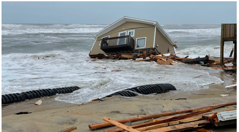
Beach homes collapsing into the ocean due to climate change have become common along the NC coast.
